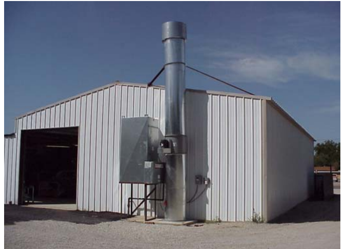
HEATER AND EXHAUST ASSEMBLY
